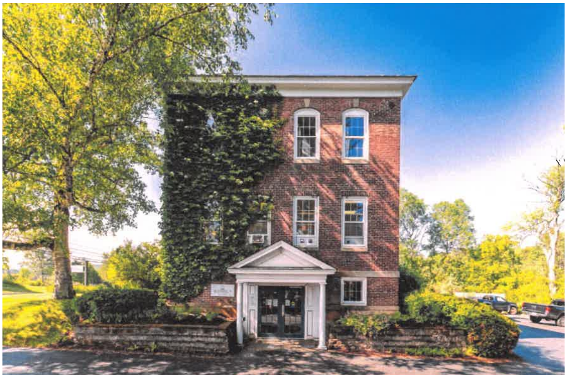
Right Side of Building
