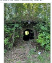
Looking East at One of the Preserved Brick Kilns.
