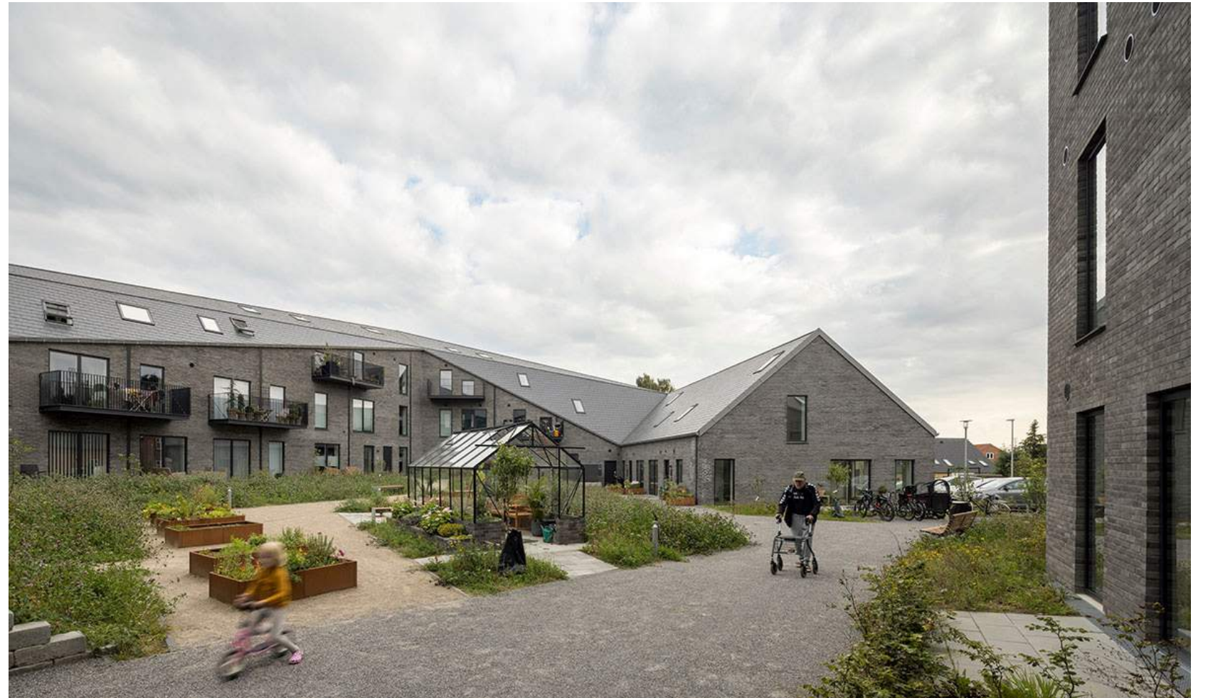
Malling Dampmølle Housing Complex, Denmark / CEBRA
