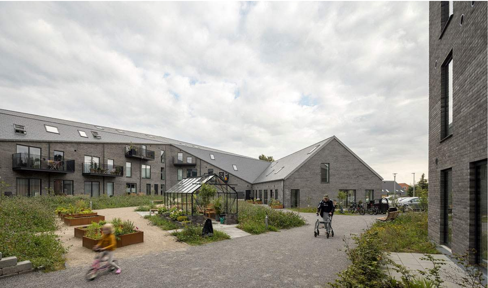
Malling Dampmølle Housing Complex, Denmark / CEBRA
