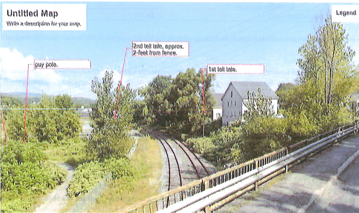
View looking north from the Route 12A Bridge (062/117)
