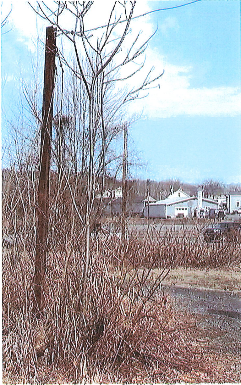
Detailed view of the steel guy pole to be removed.
