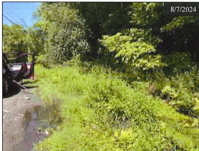
Photo 2. Route 12A northbound pull-off across from house #32 & #34 Facing north showing PEM1E foreground, PSS1Ex background Proposed impacts approximately begin in front of the parked vehicle
