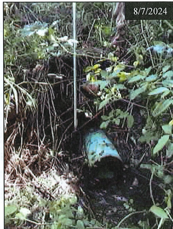
Photo 1. Road culvert outlet/wetland inlet
