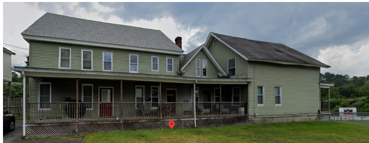
53 Water Street (5 units)
