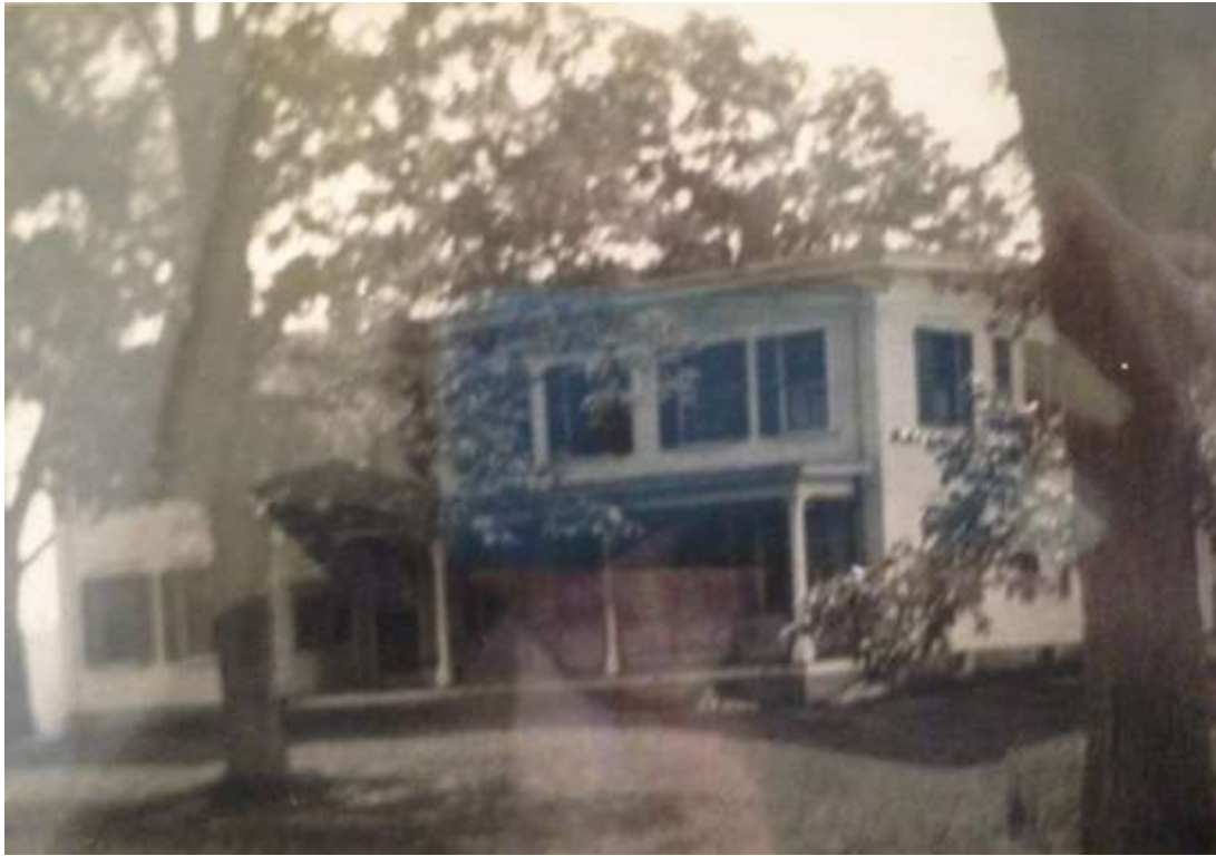
Early 20th century photo showing original front porch no longer present
