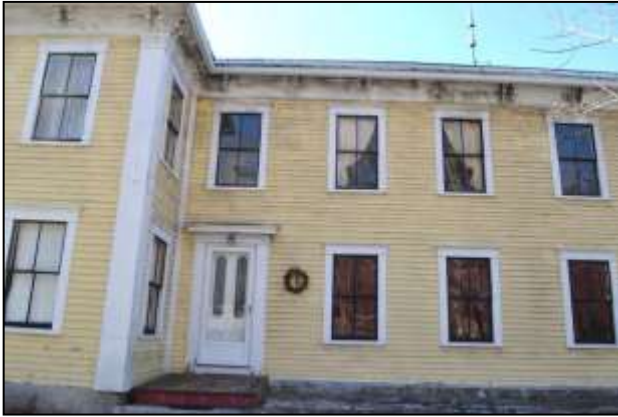
Façade (east elevation) of house, showing rear the two-light doorway, characteristic of the mid-19 th century, and casings and cornice.
