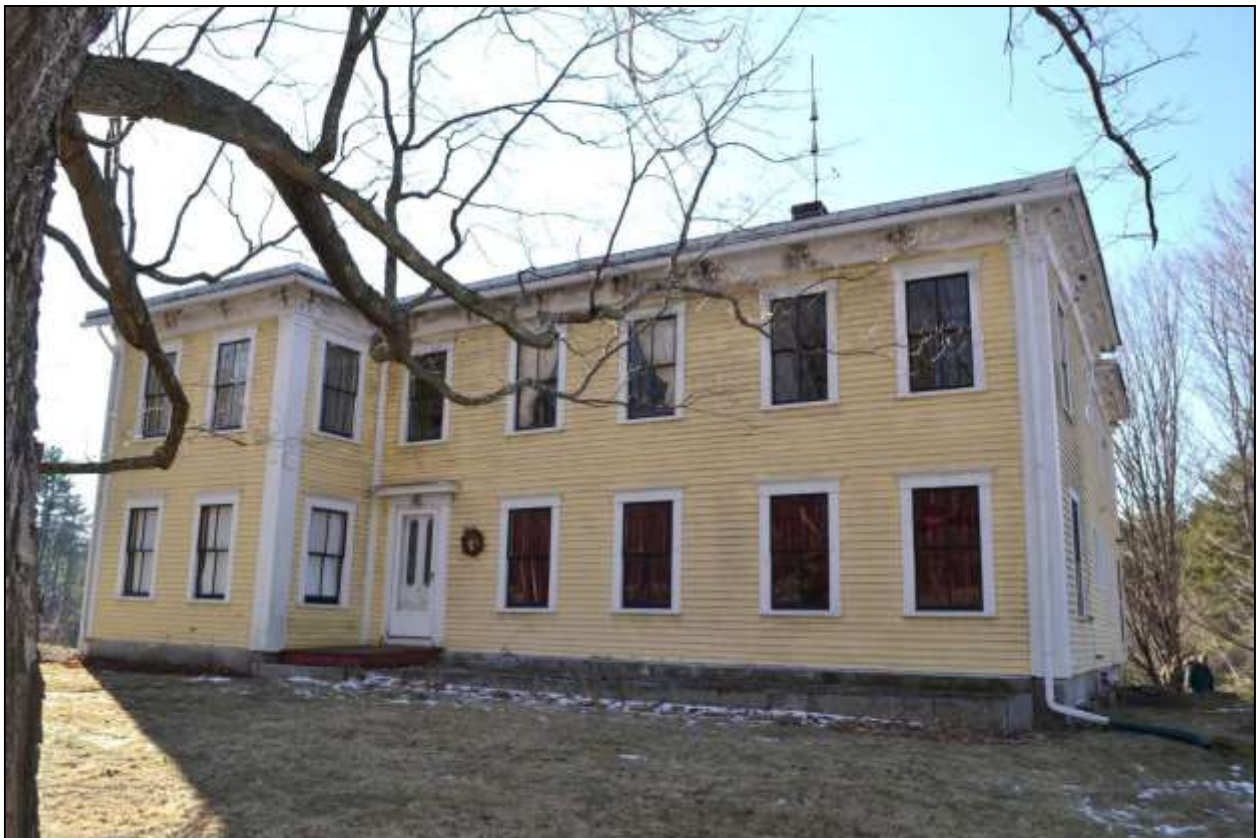
Campbell Farmhouse, North and East (Front) Elevations
