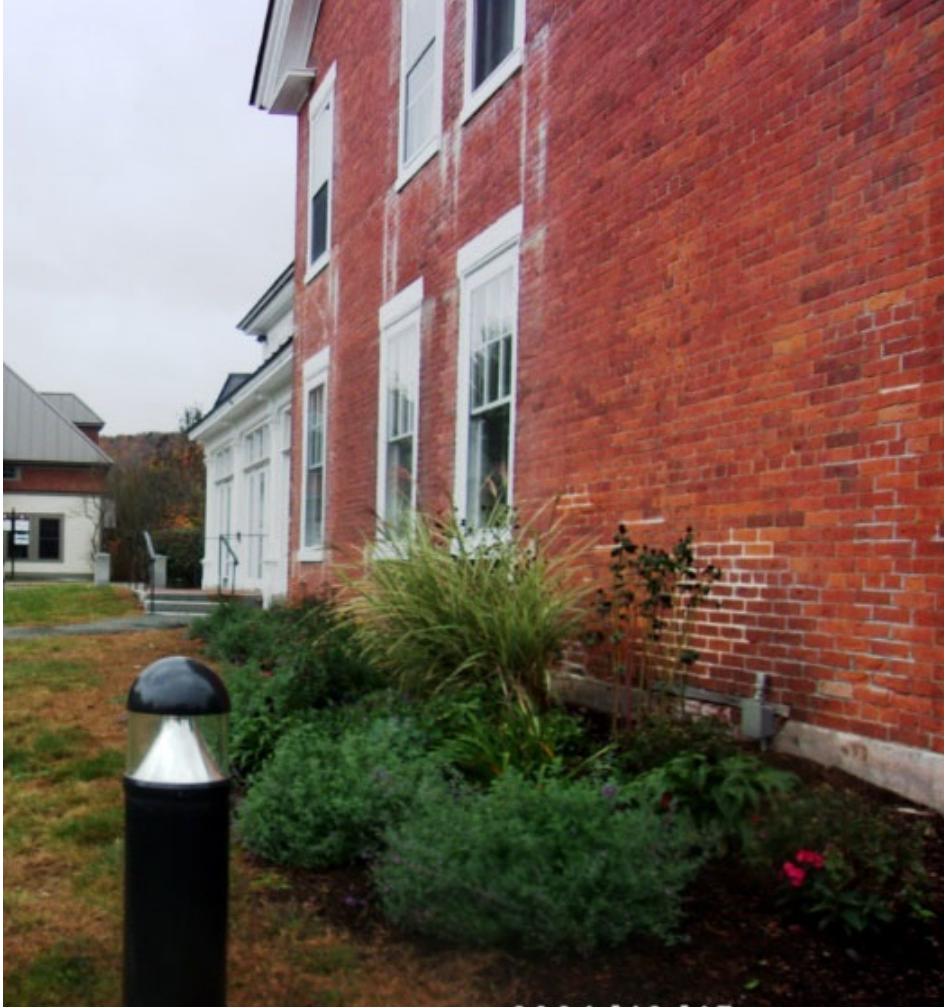
3. LOOKING SOUTH FROM ALONG EAST SIDE OF STRUCTURE
