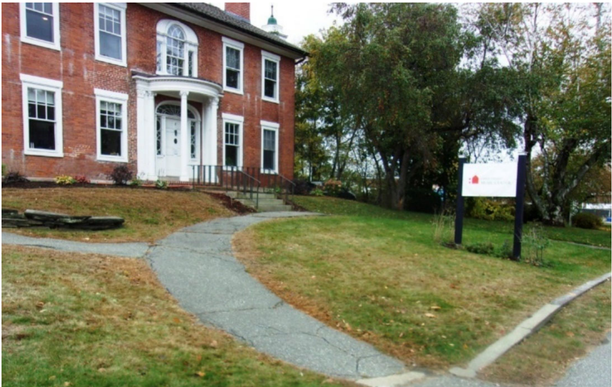
Photo 2 - LOOKING SOUTHWEST FROM SOUTH PARK STREET
