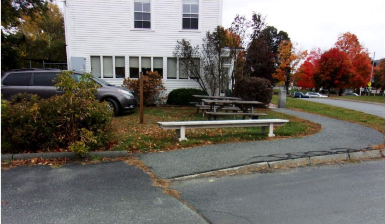
Photo 4 - LOOKING NORTH FROM REAR OF BUILDING
