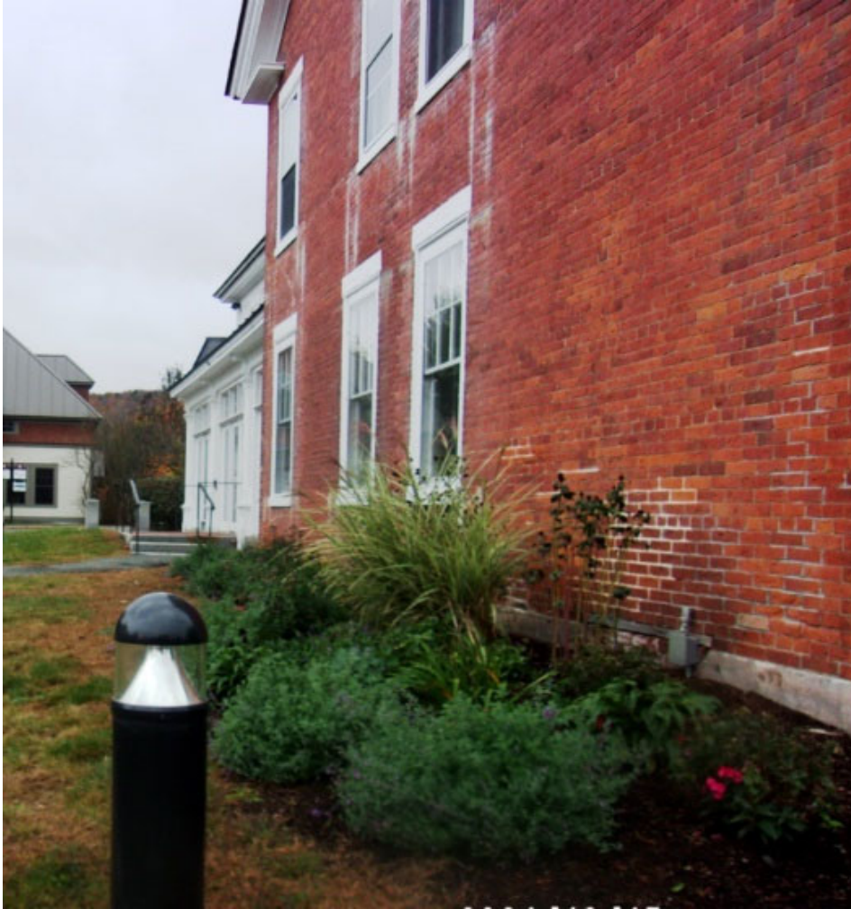
Photo 3 - LOOKING SOUTH FROM ALONG EAST SIDE OF STRUCTURE
