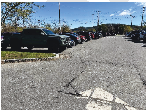
Image 11. Pavement Condition (North view)
