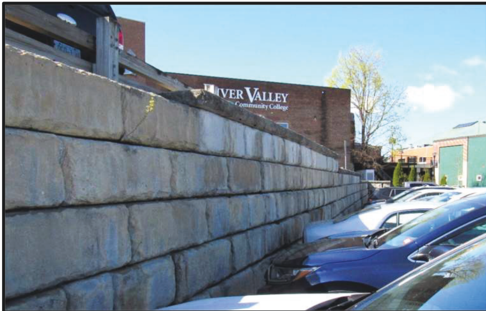
Photo 3 – General View of Wall Segment #3
