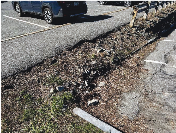
Image 7. Sidewalk/Curb Condition (South view)
