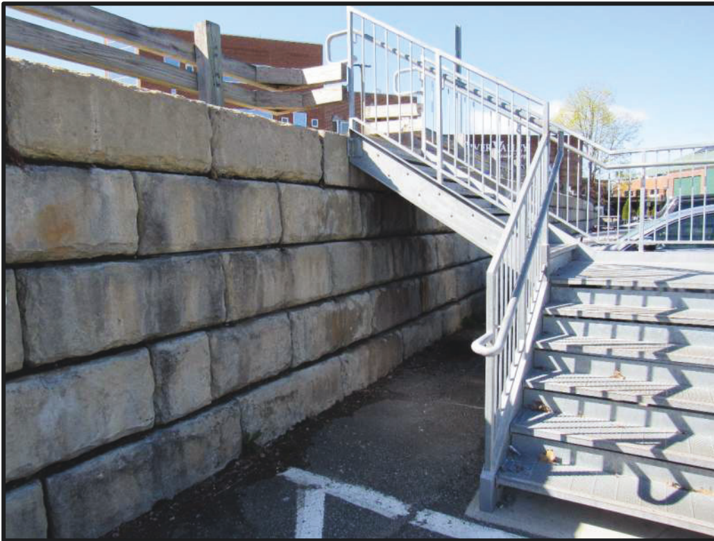
Photo 14 – Stairs Attached to Wall Segment #3
