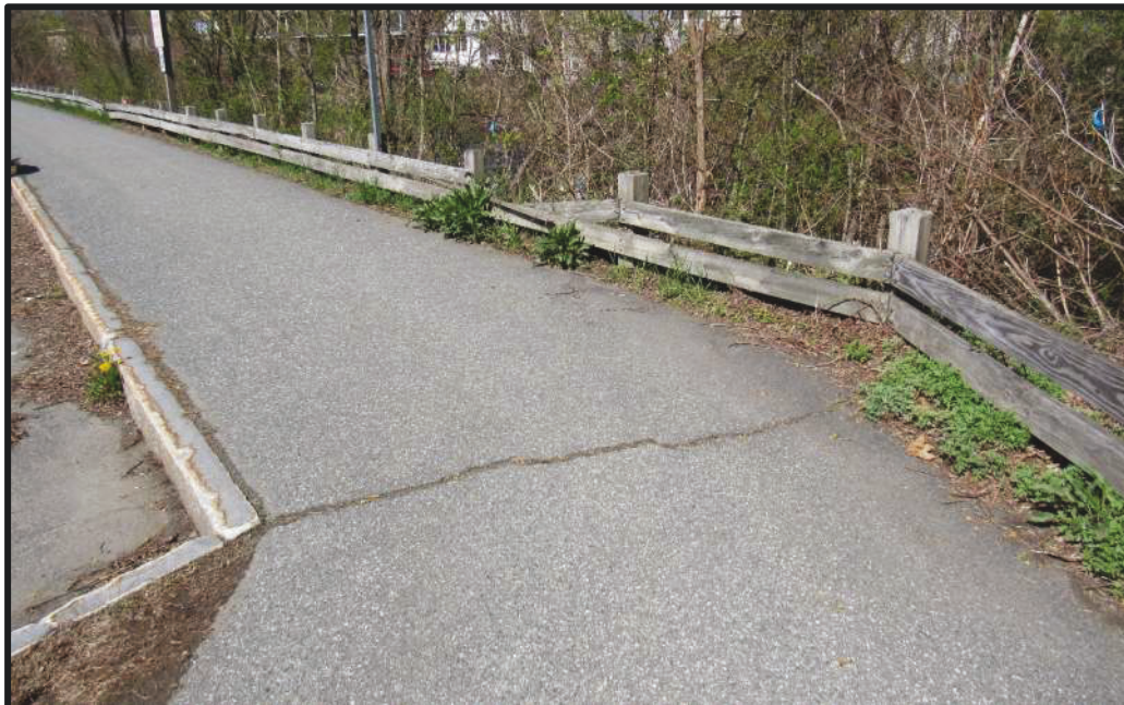
Photo 5 – General View of Guardrail Segment #2
