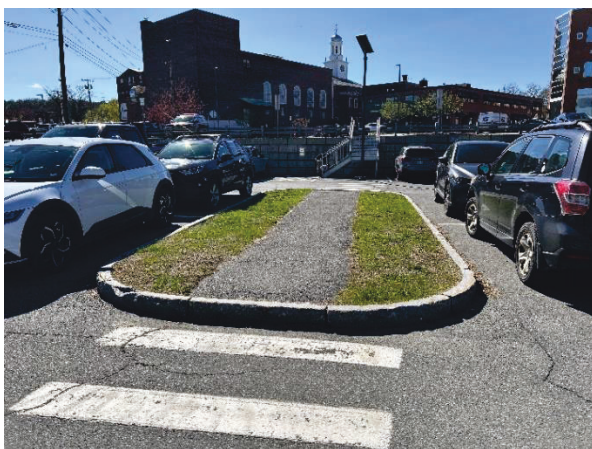
Image 3. Sidewalk Condition (Southeast View)
