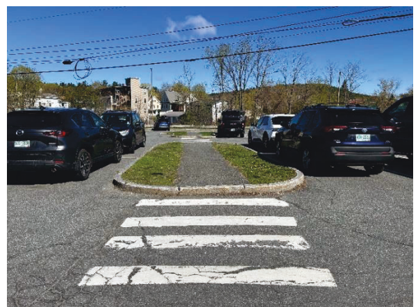
Image 6. Sidewalk Condition (Northeast View)
