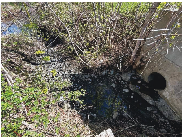
Image 12. Outlet Condition (North view)
