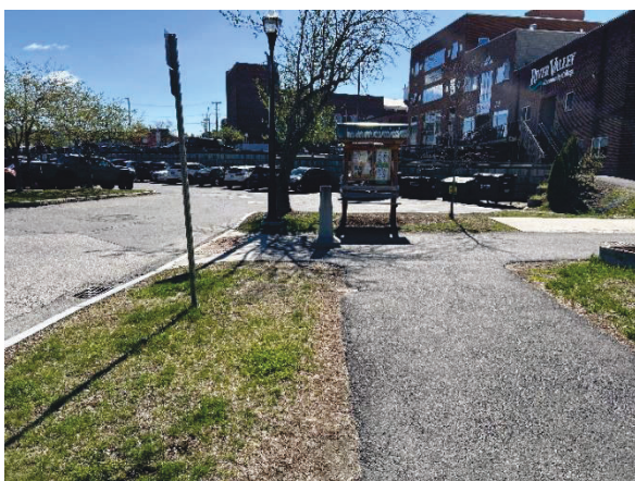
Image 5. Sidewalk Condition (Southeast view)
