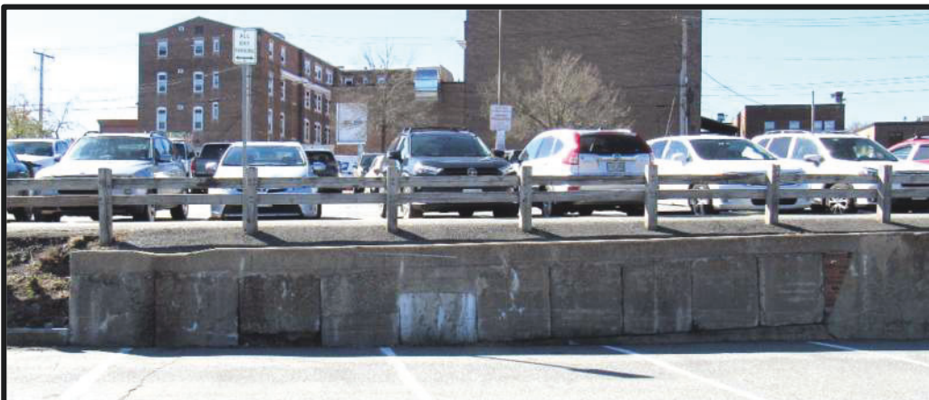
Photo 1 – General View of Wall Segment #1
