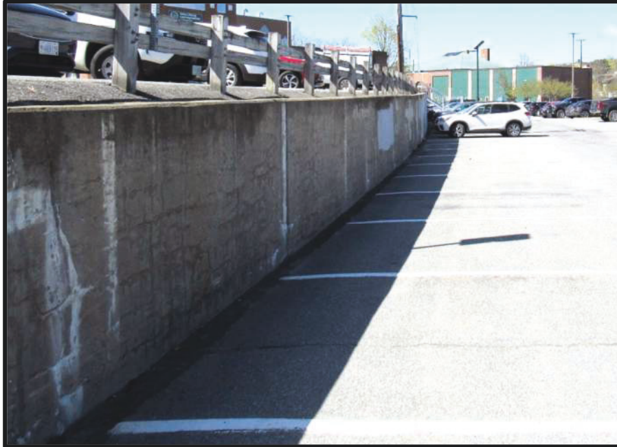
Photo 2 – General View of Wall Segment #2
