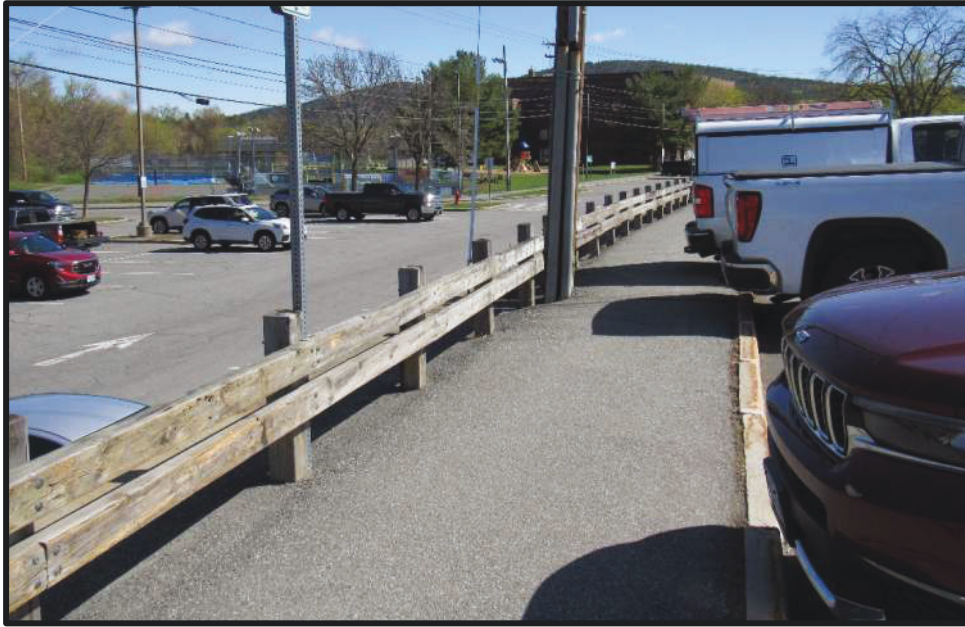
Photo 4 – General View of Guardrail Segment #1
