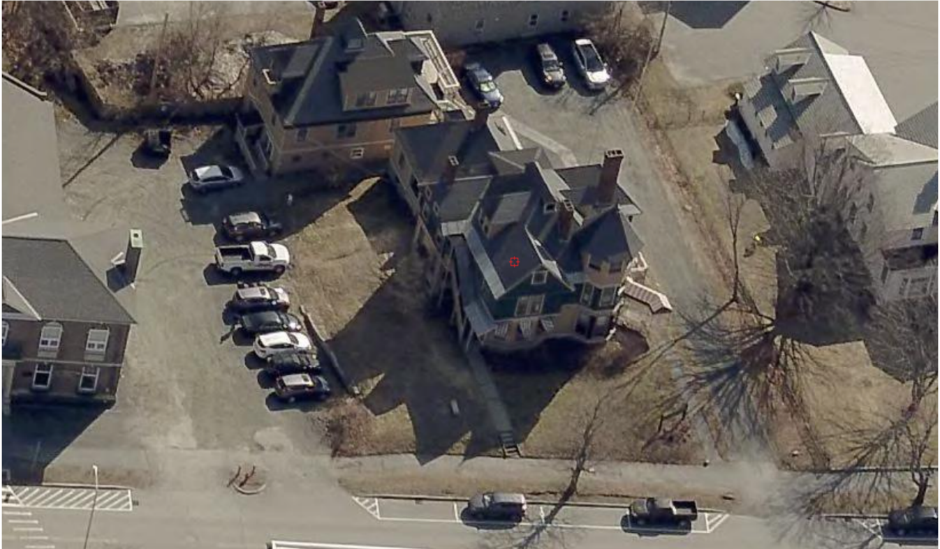
Figure 1. Bird's eye view of property (looking east).
