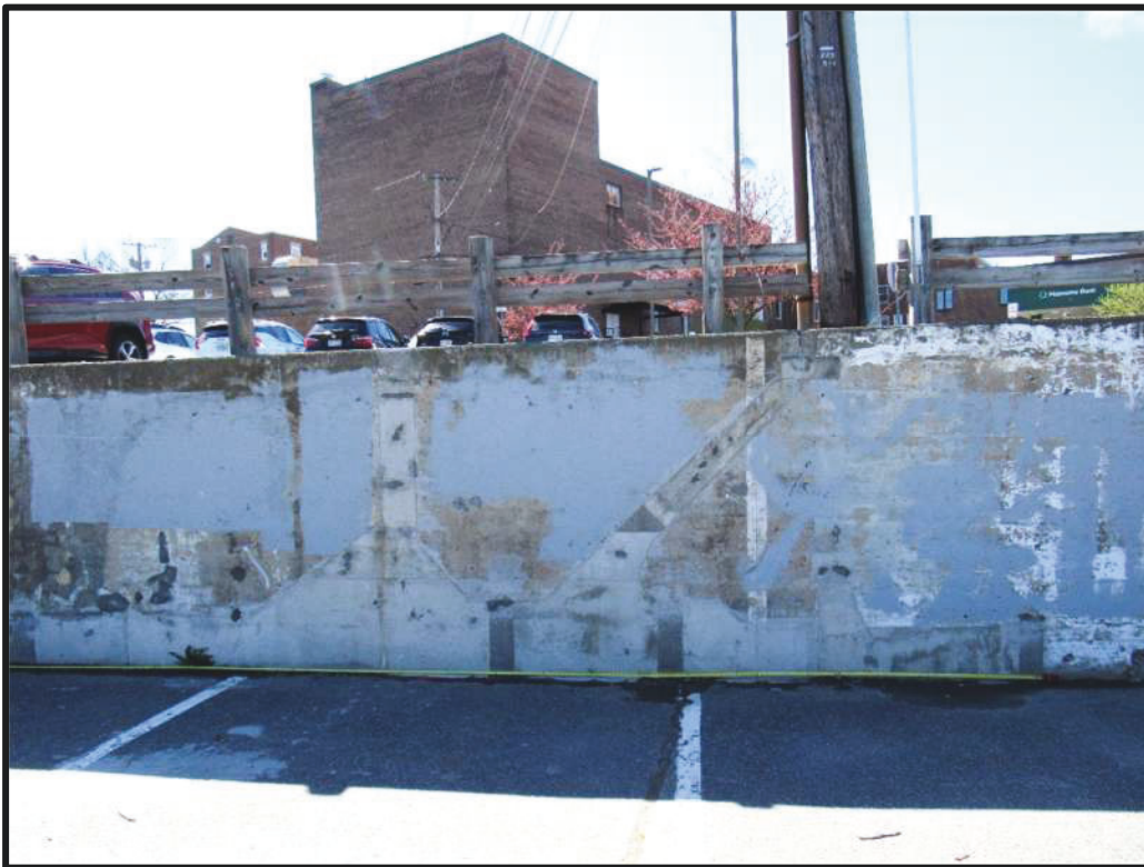
Photo 11 – Patch Repairs on Face of Wall Segment #2 Return Wall
