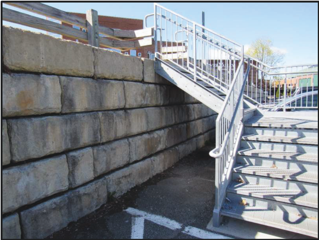
Photo 14 – Stairs Attached to Wall Segment #3
