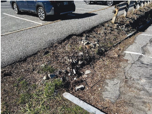
Image 7. Sidewalk/Curb Condition (South view)
