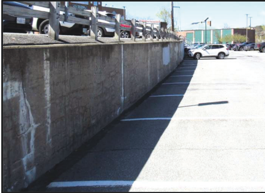
Photo 2 – General View of Wall Segment #2
