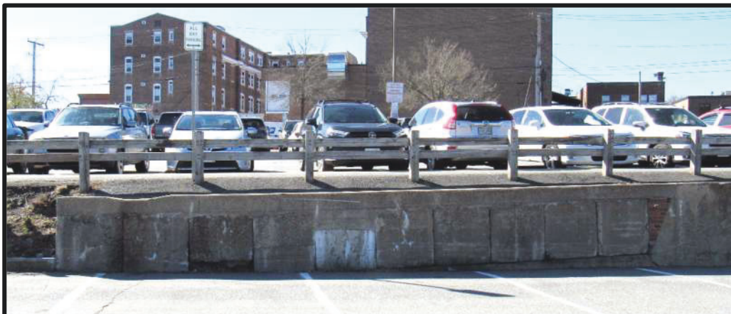
Photo 1 – General View of Wall Segment #1
