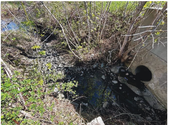
Image 12. Outlet Condition (North view)
