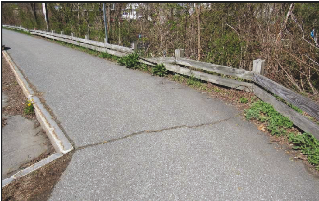
Photo 5 – General View of Guardrail Segment #2
