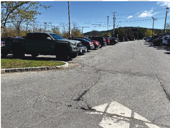
Image 11. Pavement Condition (North view)
