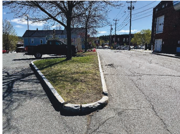
Image 8. Curb Condition (East View)
