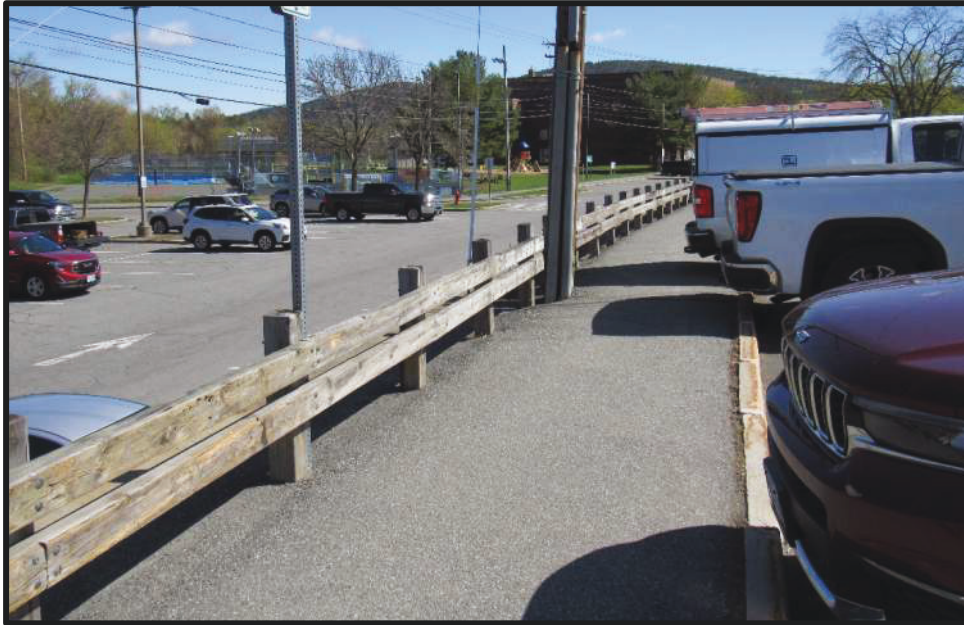
Photo 4 – General View of Guardrail Segment #1
