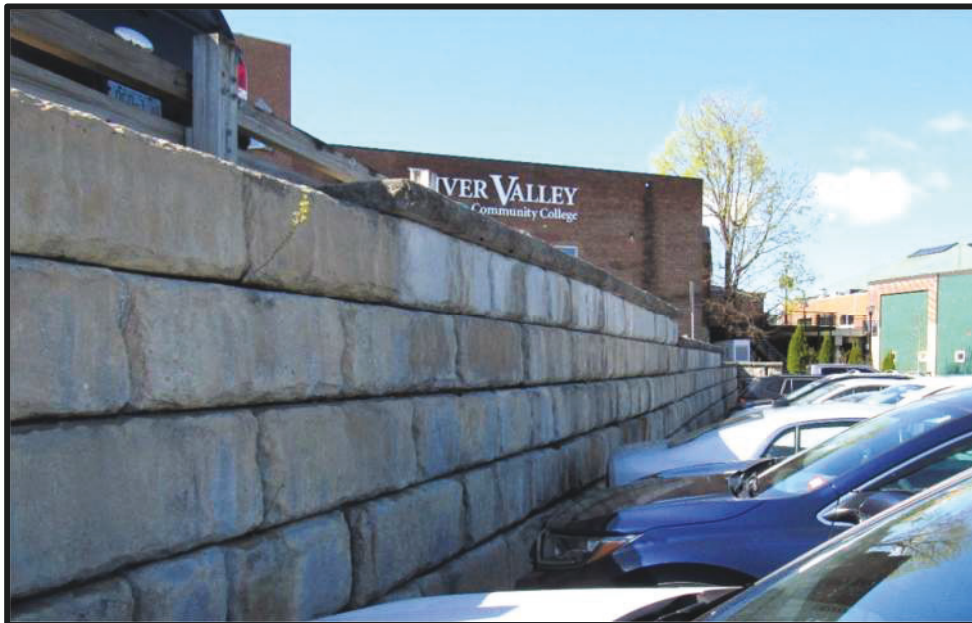
Photo 3 – General View of Wall Segment #3
