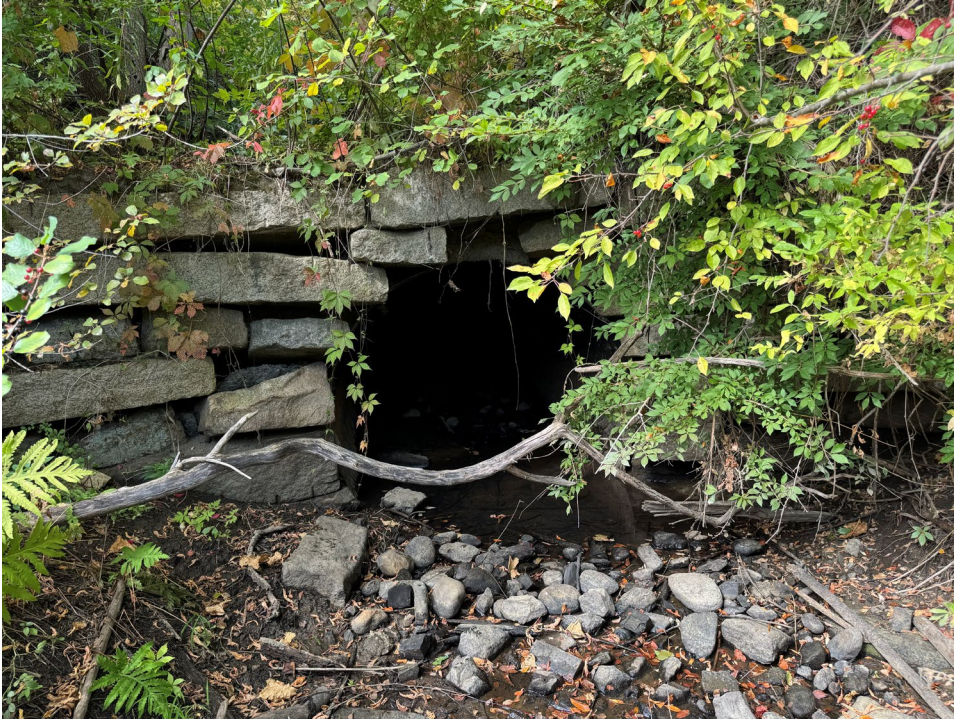
Photo 3 – Looking west, upstream at culvert outfall
