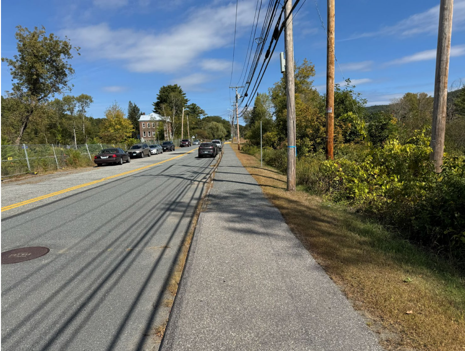
Photo 5 – Looking north on Hanover Street from culvert location
