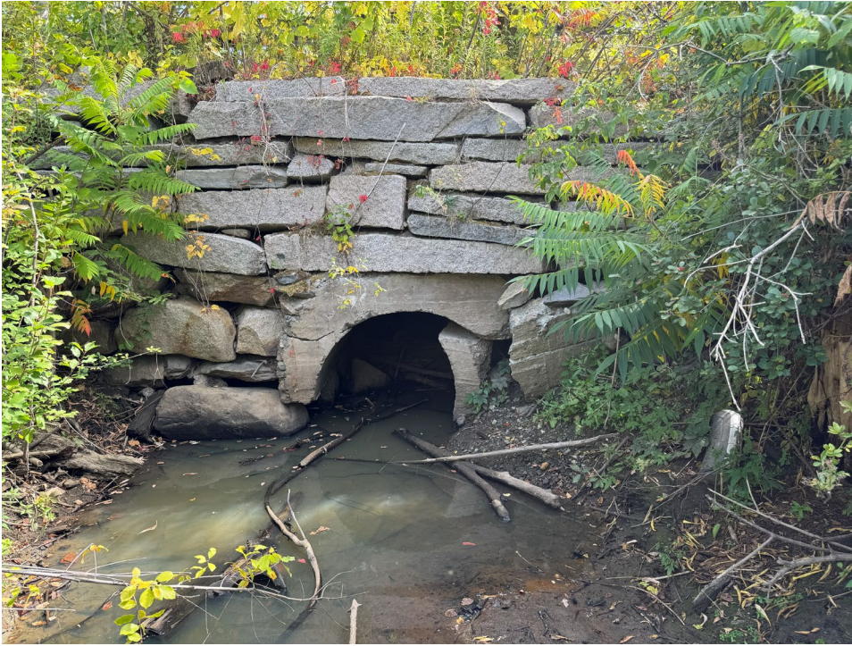
Photo 1 – Looking east, downstream towards culvert inlet
