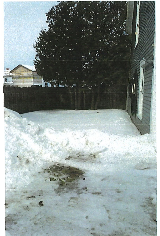
Yard behind garage where stairs are proposed
