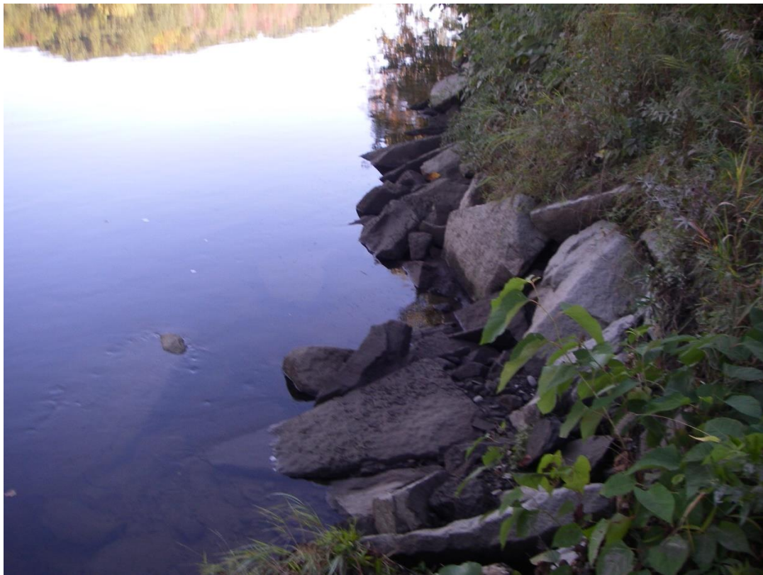
Photo 6: NH bank in northeast bridge quadrant facing north, Impact area F (09/16/2005)
