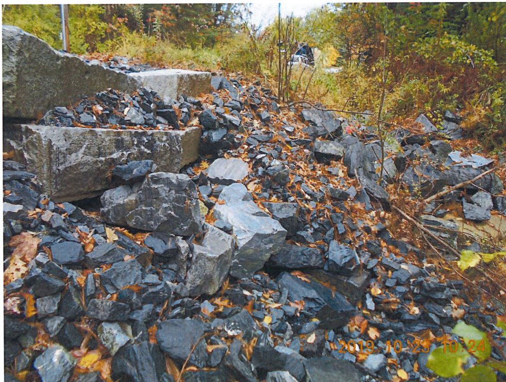
Photograph No. 6 (dated 10/23/19): View to the northwest showing the existing granite blocks and riprap on the embankment above the existing 24" culvert.
