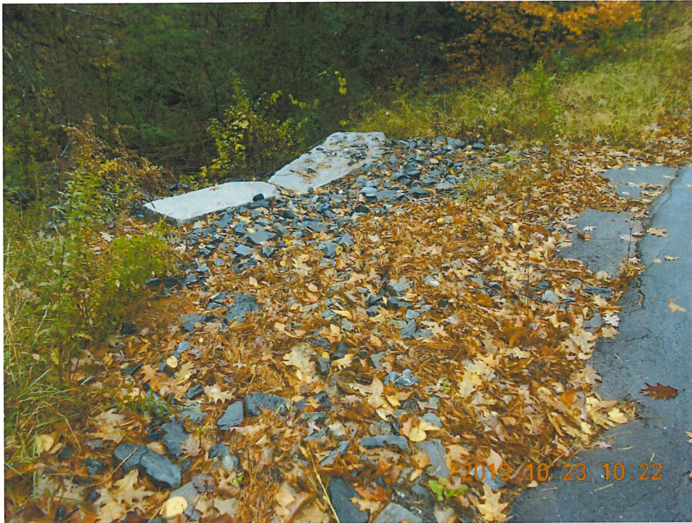
Photograph No. 5 (dated 10/23/19): View to the south from the roadway showing the existing granite blocks and riprap on the embankment above the existing 24" culvert.
