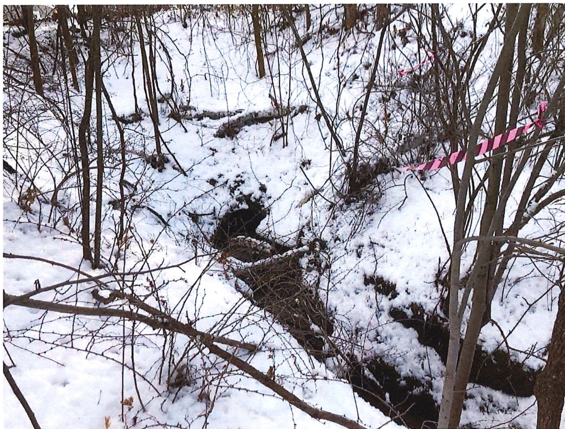
Photograph 1: Existing stormwater outfall
