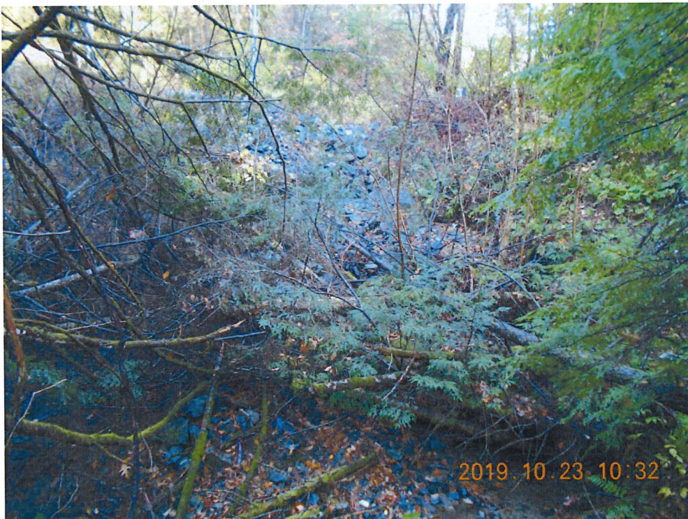
Photograph No. 14 (dated 10/23/19): View to the northeast from the down-gradient end of the project area showing the tree debris clogging the ravine.
