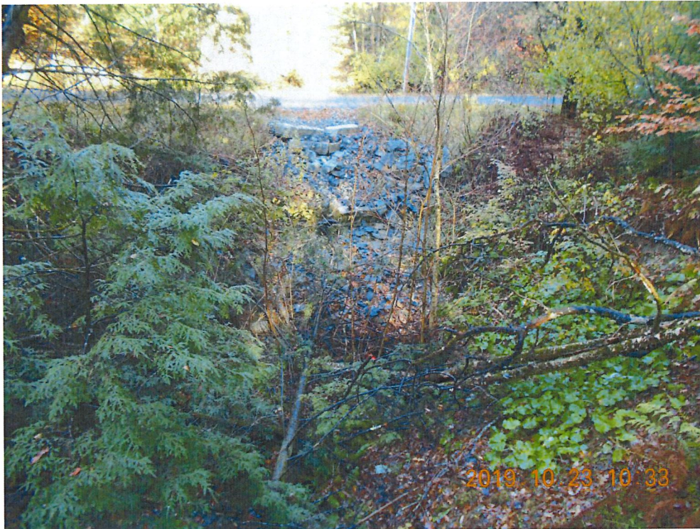
Photograph No. 13 (dated 10/23/19): View to the northwest from the bank opposite of the road showing the riprap on the embankment slopes and tree debris in the ravine.
