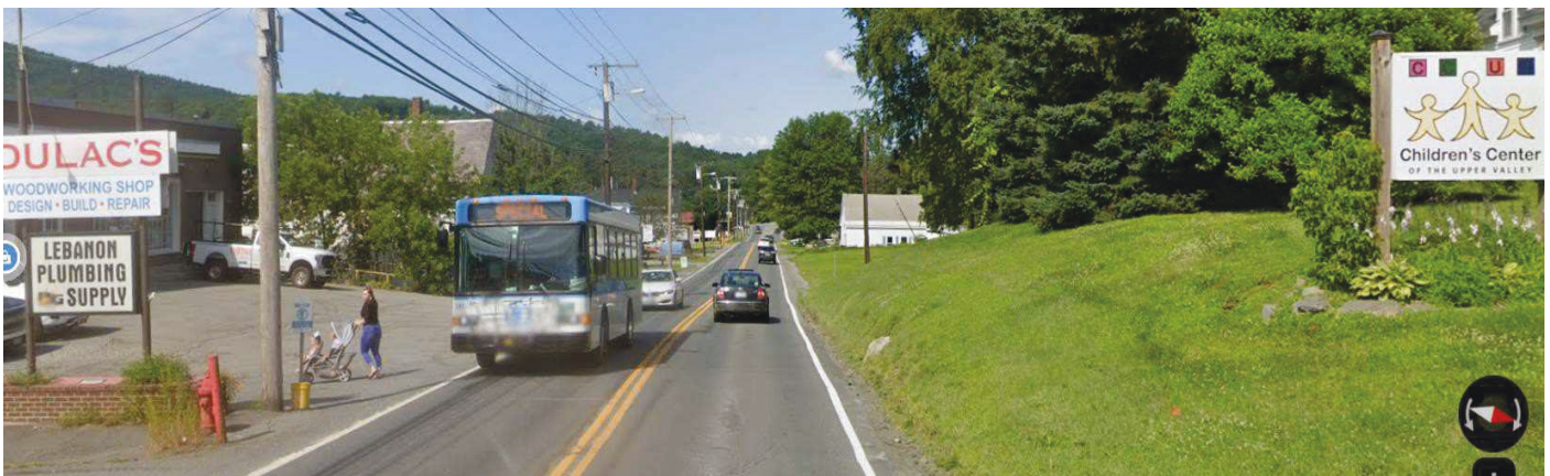
Photo of pedestrian and Advance Transit on Mechanic Street, east of the subject project area, demonstrating the narrow roadway and lack of safe space for pedestrians/transit users.
