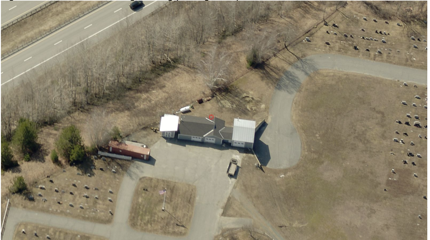
Figure 1. Aerial View of Existing Building ( looking south ).
