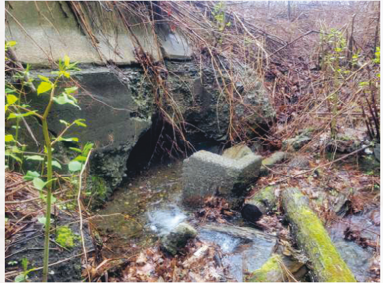
Upstream End of Culvert
