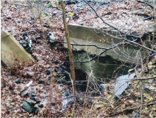
Downstream End of Culvert
