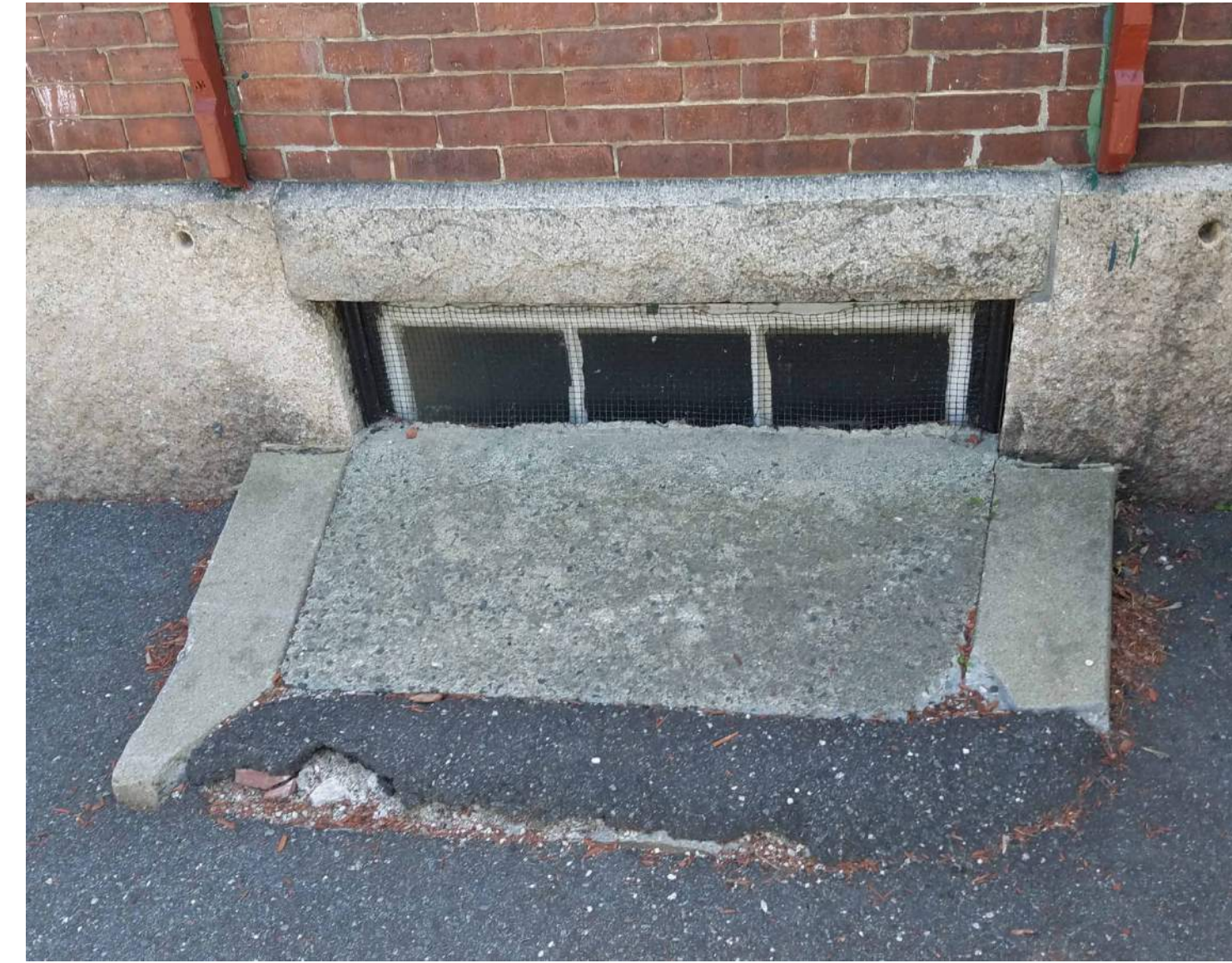
TYPICAL WINDOW WELL TO BE OPENED UP
