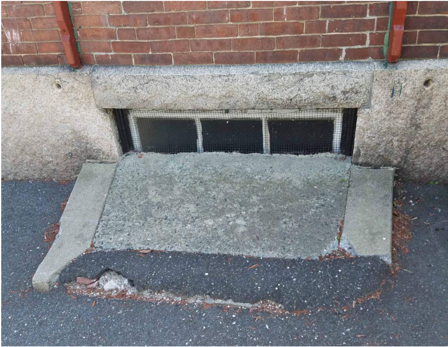
TYPICAL WINDOW WELL TO BE OPENED UP
