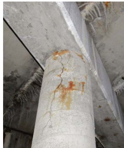
Figure 2.4 – Column splitting
