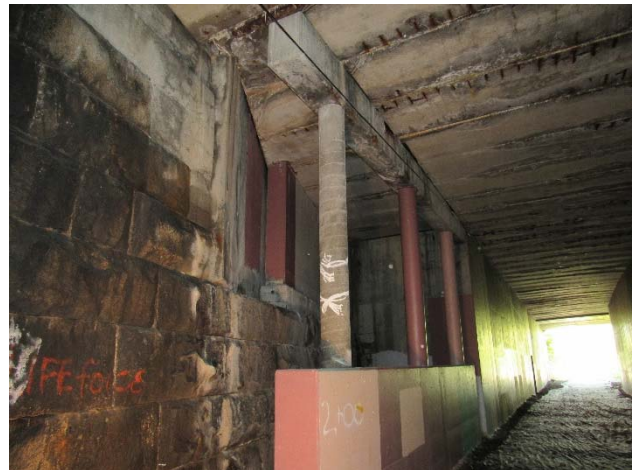
Figure 1.5 –View of pier looking south
