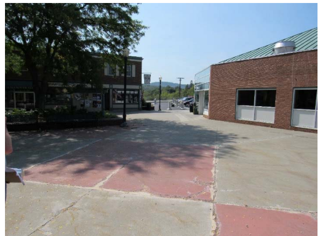
Figure 1.4 –View of plaza looking southwest
