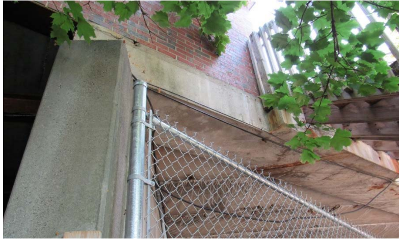
Figure 2.5 – Building partially supported on superstructure
