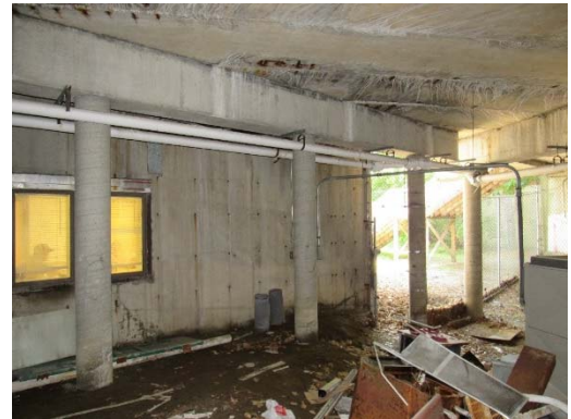
Figure 4.3 –Window near east end of tunnel
