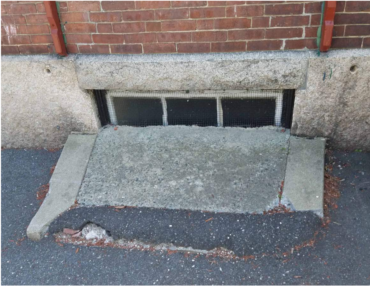
TYPICAL WINDOW WELL TO BE OPENED UP
