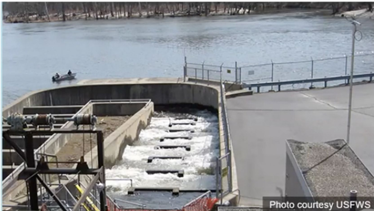
Fish Ladder, Vernon dam
