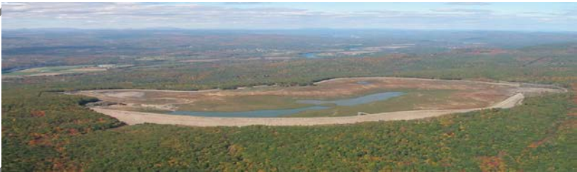
Northfield Mtn Pumped Storage
