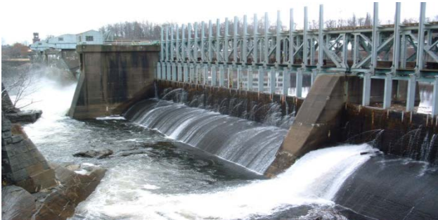
Bellows Falls Dam
