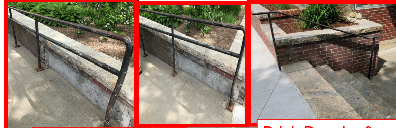
Metal Rail Repairs and repainting
