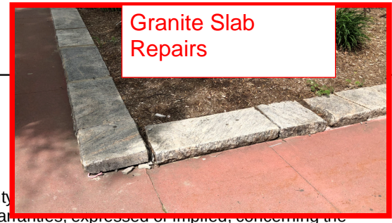
Granite Slab Repairs
