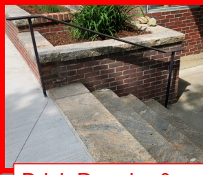
Brick Repairs & Repointing
