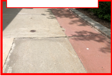
Mosaic Tile Repairs
